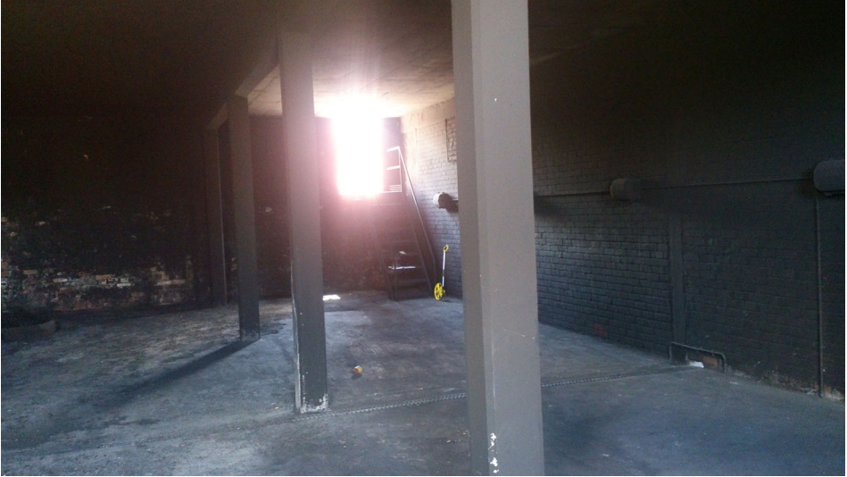
Figure 2. Inside the live fire training structure, facing the front of the structure.
