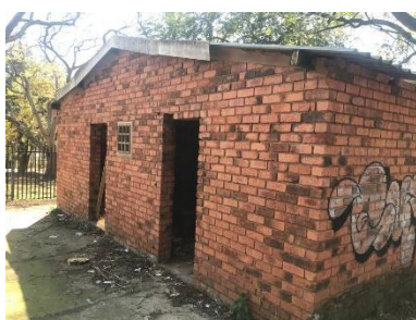
a. Alexandra Park ablution building
