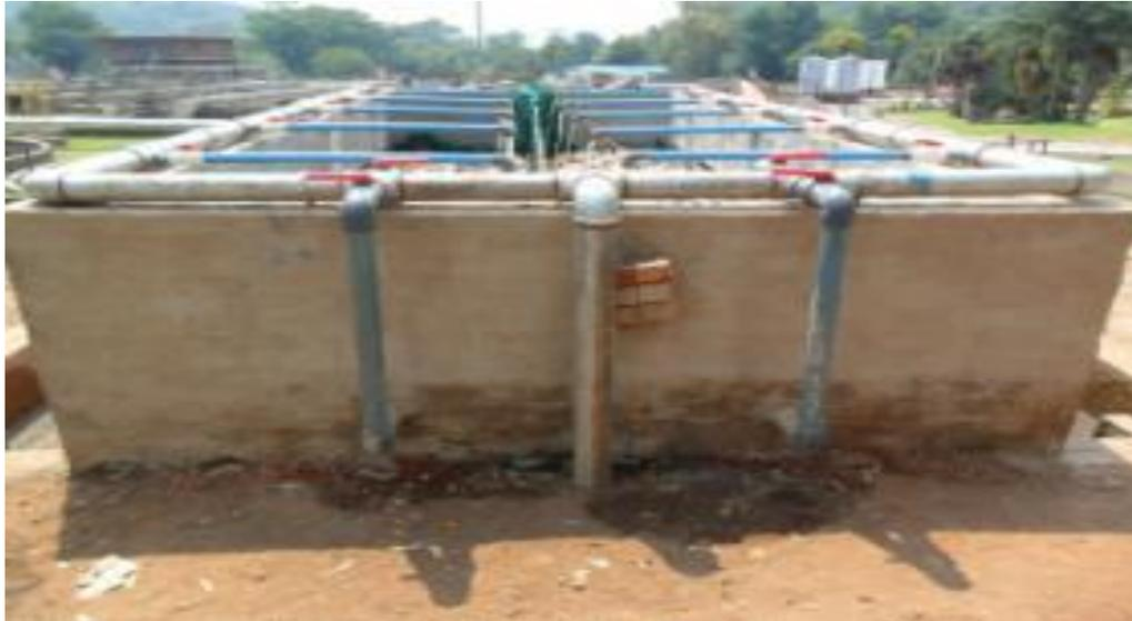
**Figure 3.** Front view of the multi-engineered system. The middle vertical pipe comes from the tank. The vertical pipes on the left and right are the pipes to the bottom inlet for subsurface flow. Small pipes on top of the bed along the wetland are for vertical flow, while those of surface flow are at the inside front of the system.
