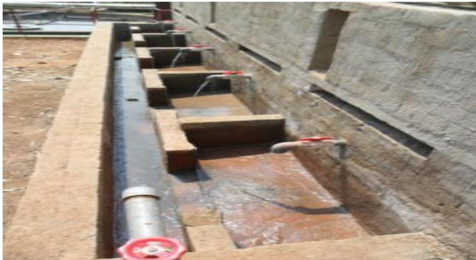
**Figure 4.** Basins and waste channel with a bypass outlet option in the left hand bottom corner of the multi-engineered system constructed at Kingsburgh, Durban.
