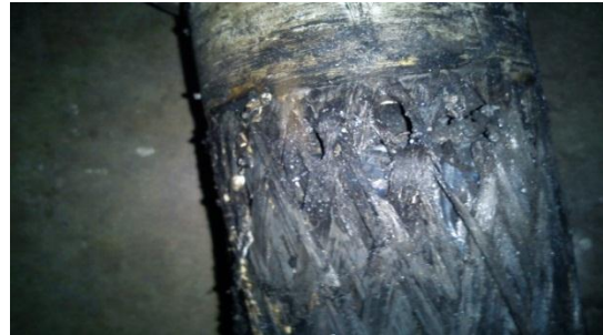
Figure 18. Damp on zinc oxide varistors.
