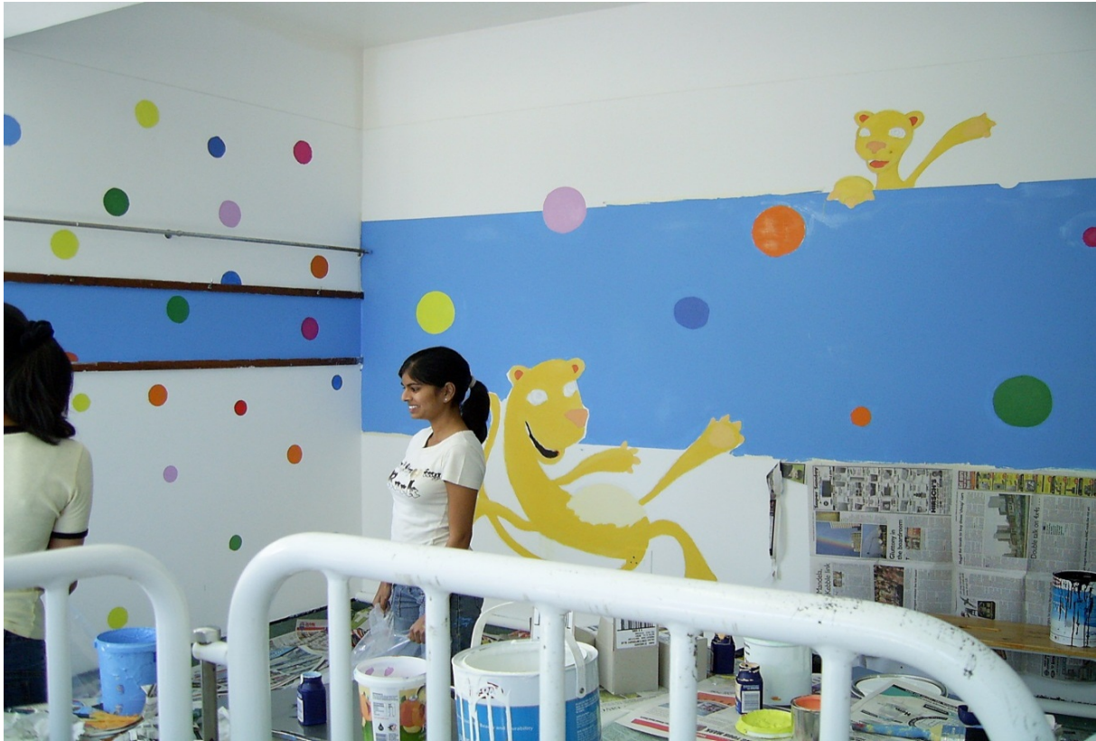
Figure 4(b). Renovating of the paediatric ward.
