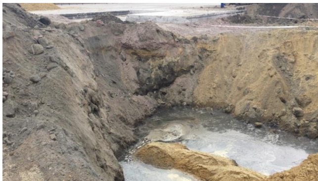
Figure 15: Rubble used as backfill
