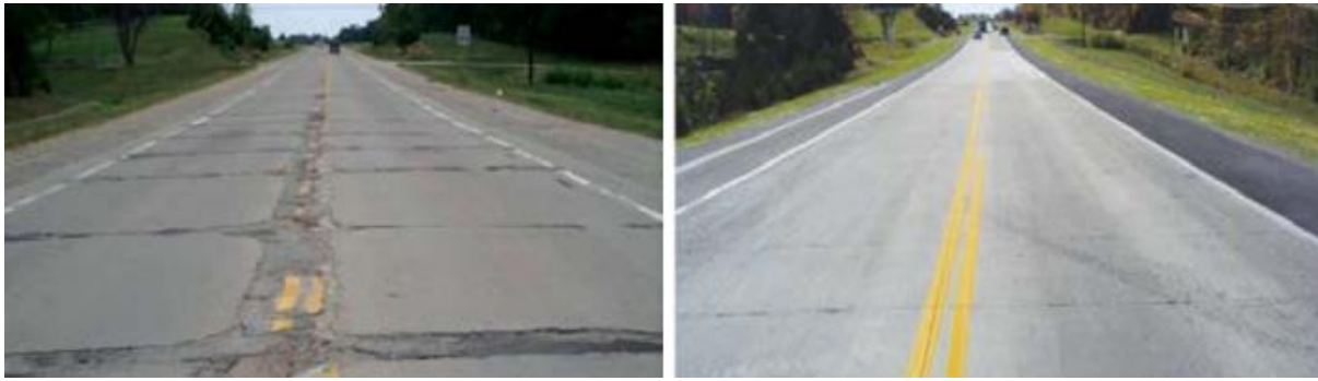
Figure 1: Typical concrete overlay (before [left] and after concrete overlay placement [right])
