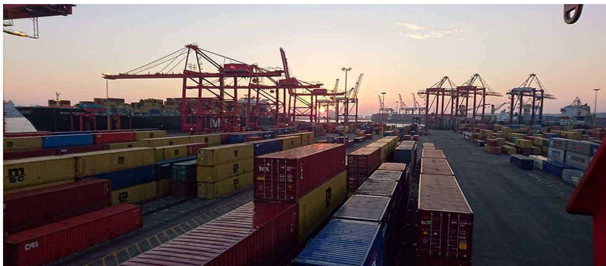
Figure 1.1: Durban Container Terminal (DCT) Pier 2 – Transnet Durban Port
